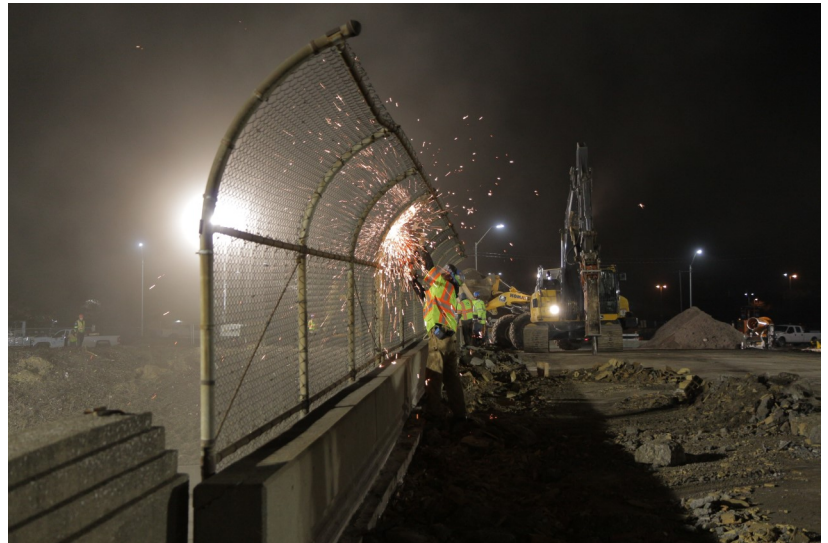
Demolition of the Chene Street bridge.
